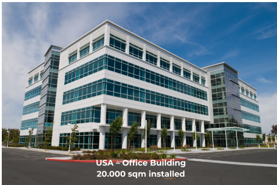
USA Office Building Ceramic tile 60 x 60 cm x 9 mm Metal raised access floor Floor q.ty 20.000 sqm
